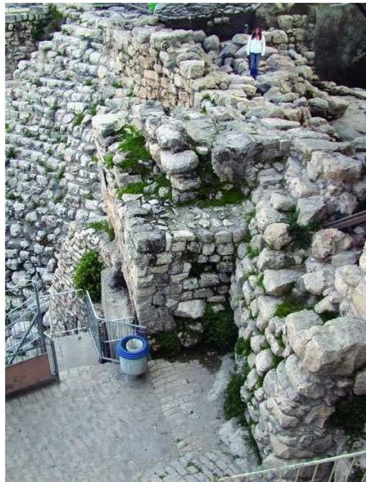
historical portion of Nehemiah's wall. You can see how broad the base is and each individual layer. The base had to be able to support the weight of the wall, while its width added strength and stability.
